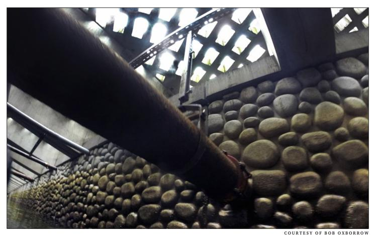
The new Seattle seawall was designed to help juvenile salmon survive. Its wall structures and underwater shelves are built with cobbled textures that are helpful to salmon and organisms they eat. For instance, the overhead walkway is a light-penetrating surface made with blocks of glass because juvenile salmon prefer swimming and eating in sunlight.
