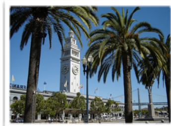
Embarcadero and Ferry Terminal Building
