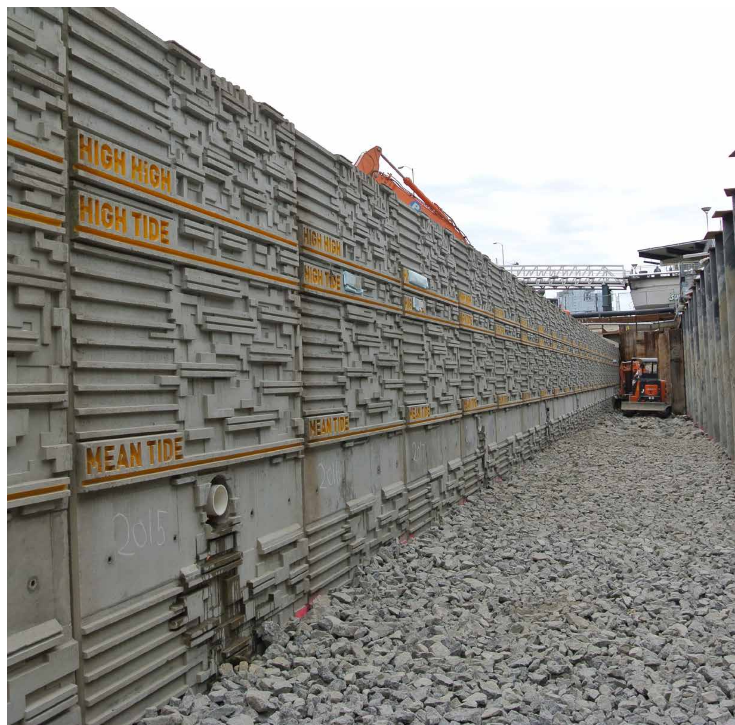
The textured seawall face provides a place for vegetation and invertebrates to grow.
