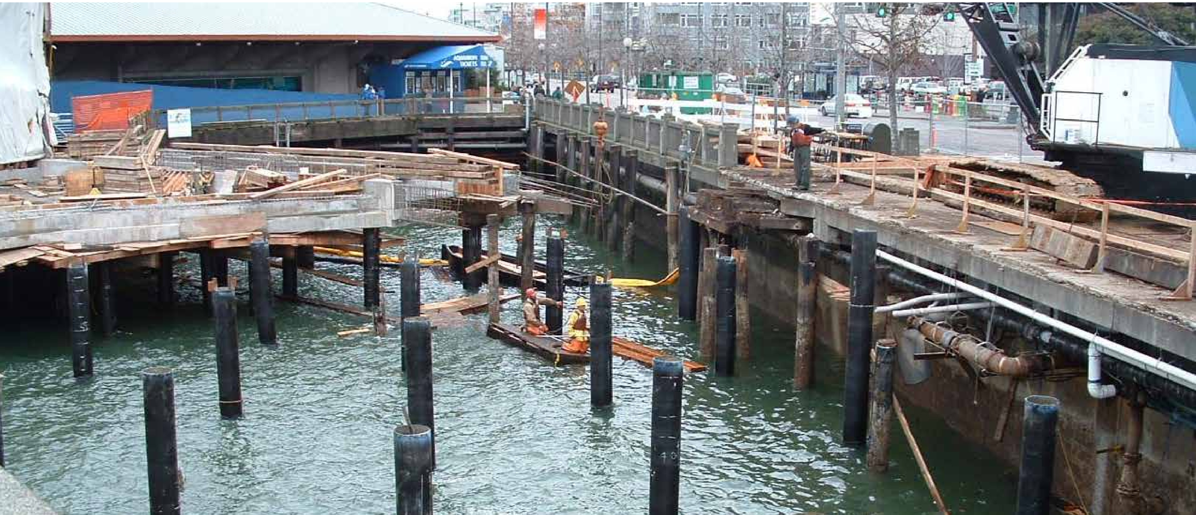
The 2005 rebuild of Pier 59 used similar construction methods. This photo was taken after the new steel piles were installed.
