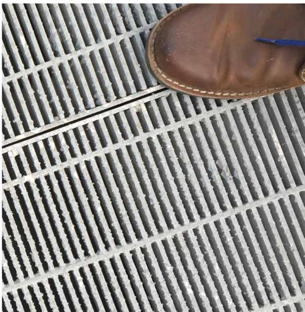
Metal grating provides additional light to nearshore habitat along the seawall.
