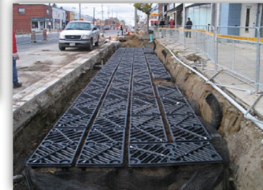
Pictured at left is the base of Silva Cells. Pictured at right are the top of the Silva Cells and base for sidewalk.
