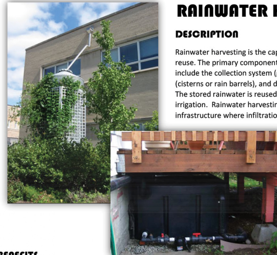
Pictured at left is a cistern with a planted trellis that receives runoff from the rooftop. Pictured at center is a cistern installed under a deck.
