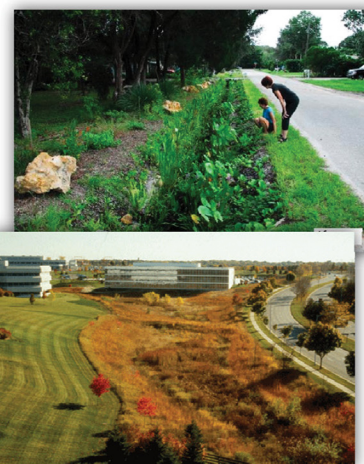
Pictured at the top is a biofiltration swale that receives runoff from a street. The lower picture shows a biofiltration swale that receives runoff from a sidewalk and office park.
